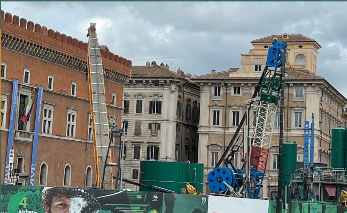
Construction work for the metro line in the historic center of Rome, Italy. © RERM
